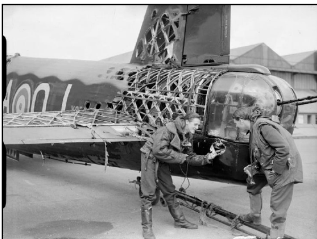
Wellington Bomber WW2, showing the vulnerability of the rear gunner position and thin air frame
